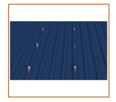
Step 2: Install all U Mini rail on metal sheet roof .
